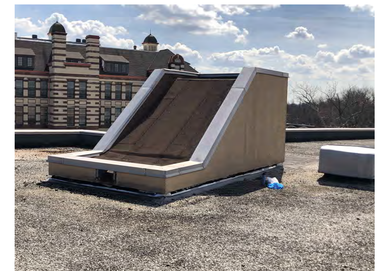
PHOTO # 24 - STAIR TOWER ROOF
