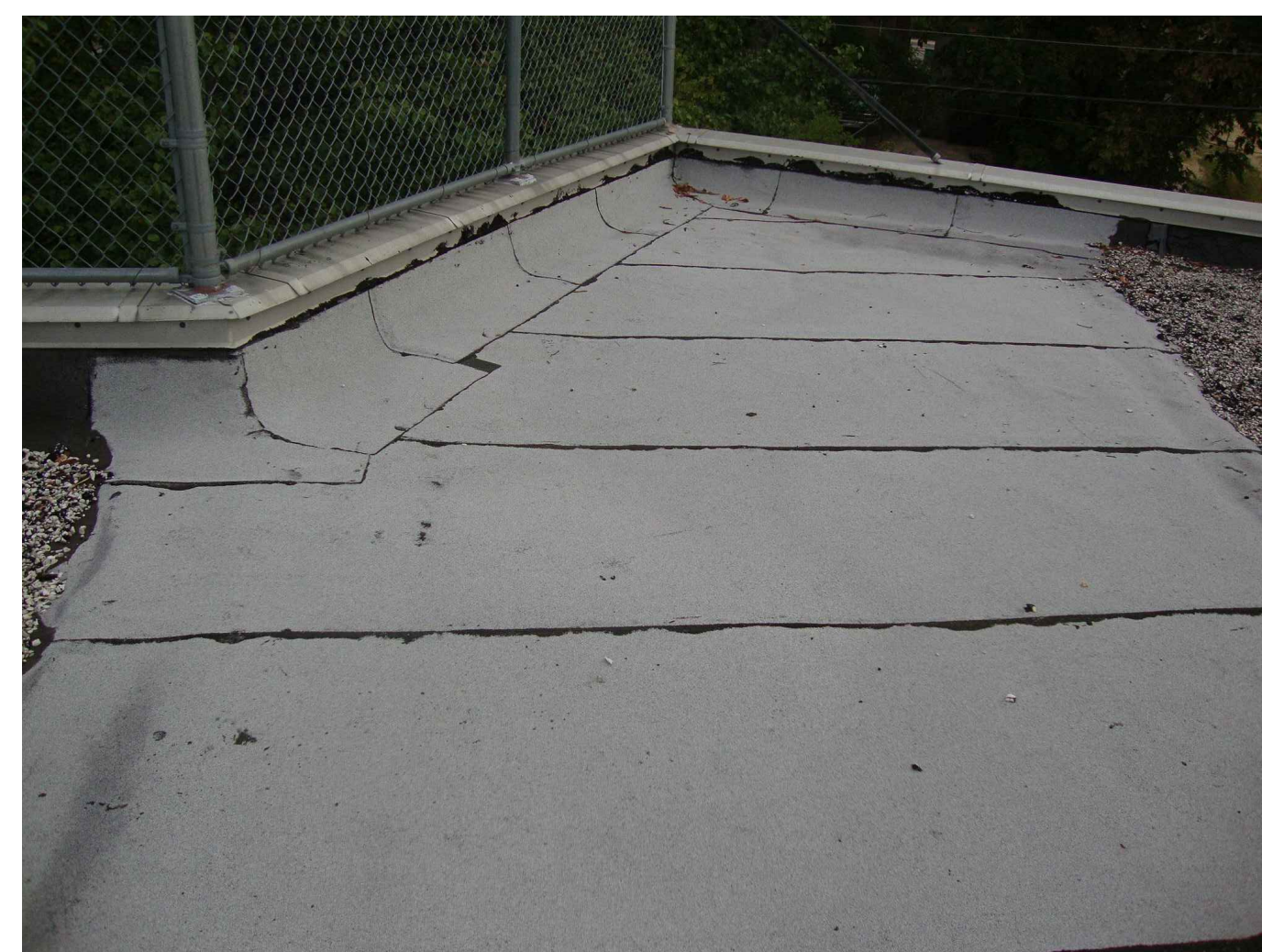
PHOTO # 22 - MAIN ROOF PARAPET AT FENCE
