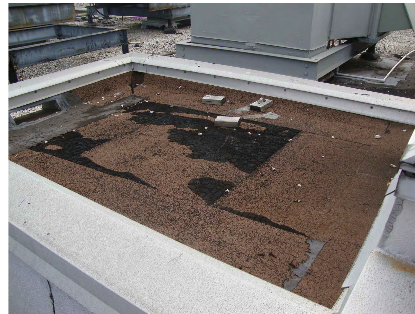
PHOTO # 19 - ELEVATOR ROOF
