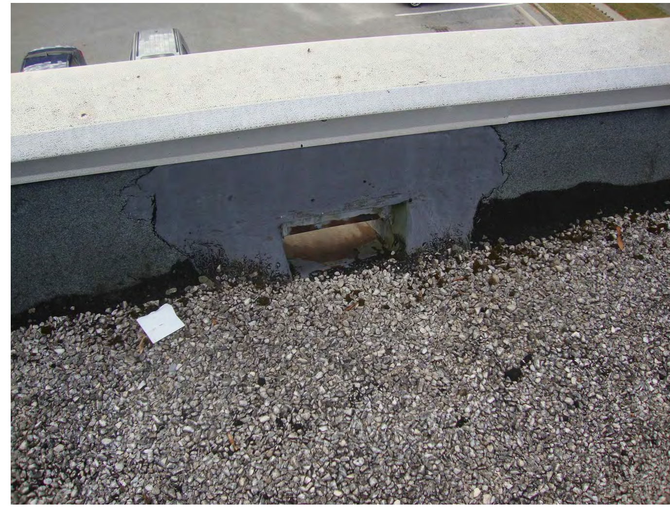
PHOTO # 27 - THROUGH WALL SCUPPER
