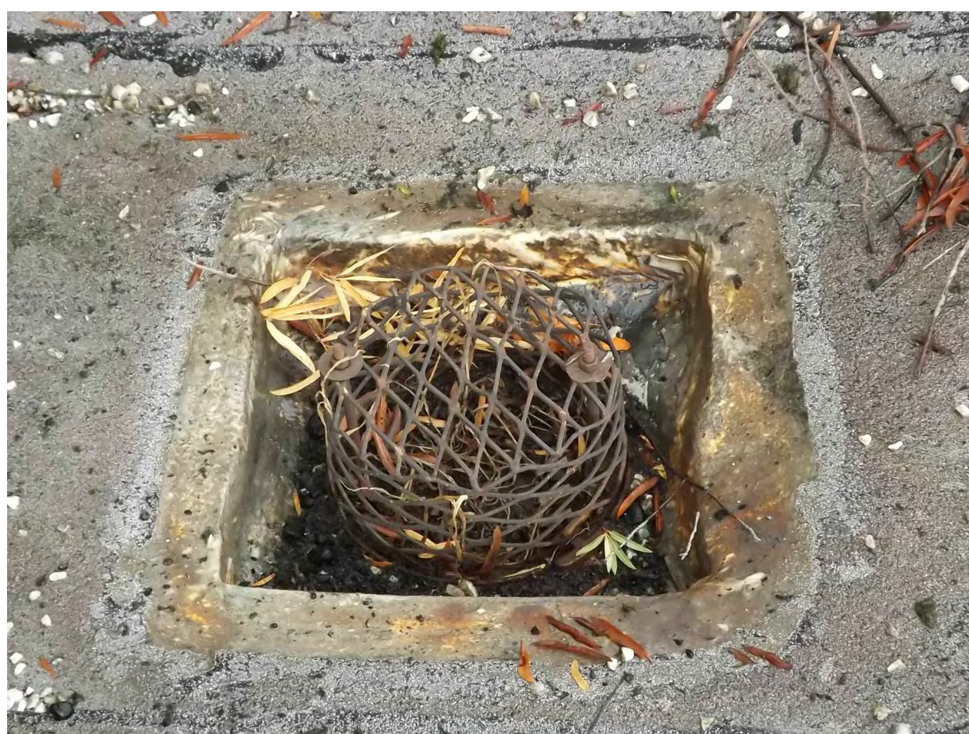
PHOTO # 33 - ROOF DRAIN ON MAIN ROOF
