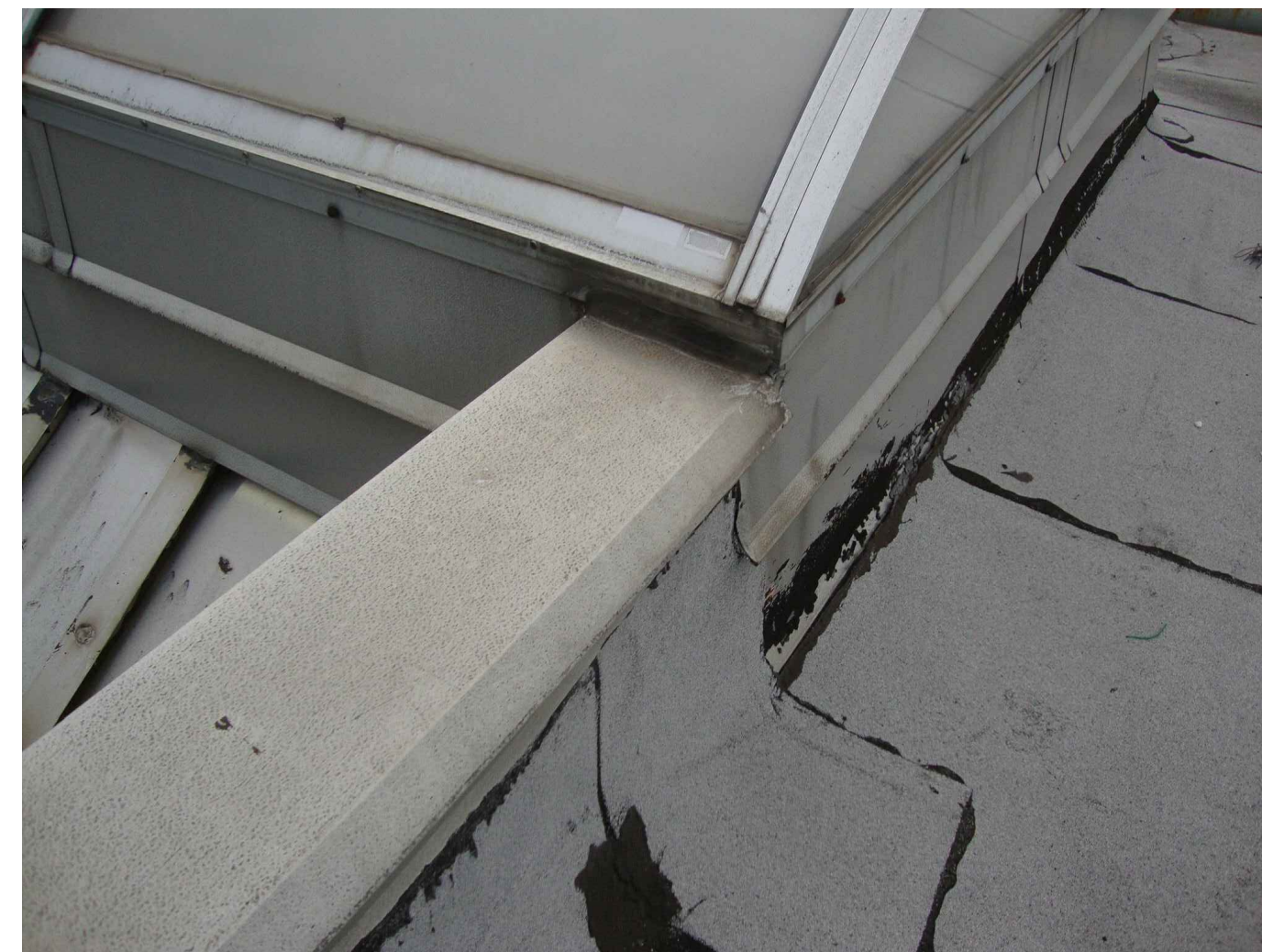
PHOTO # 18 - PARAPET/SKYLIGHT TRANSITION
