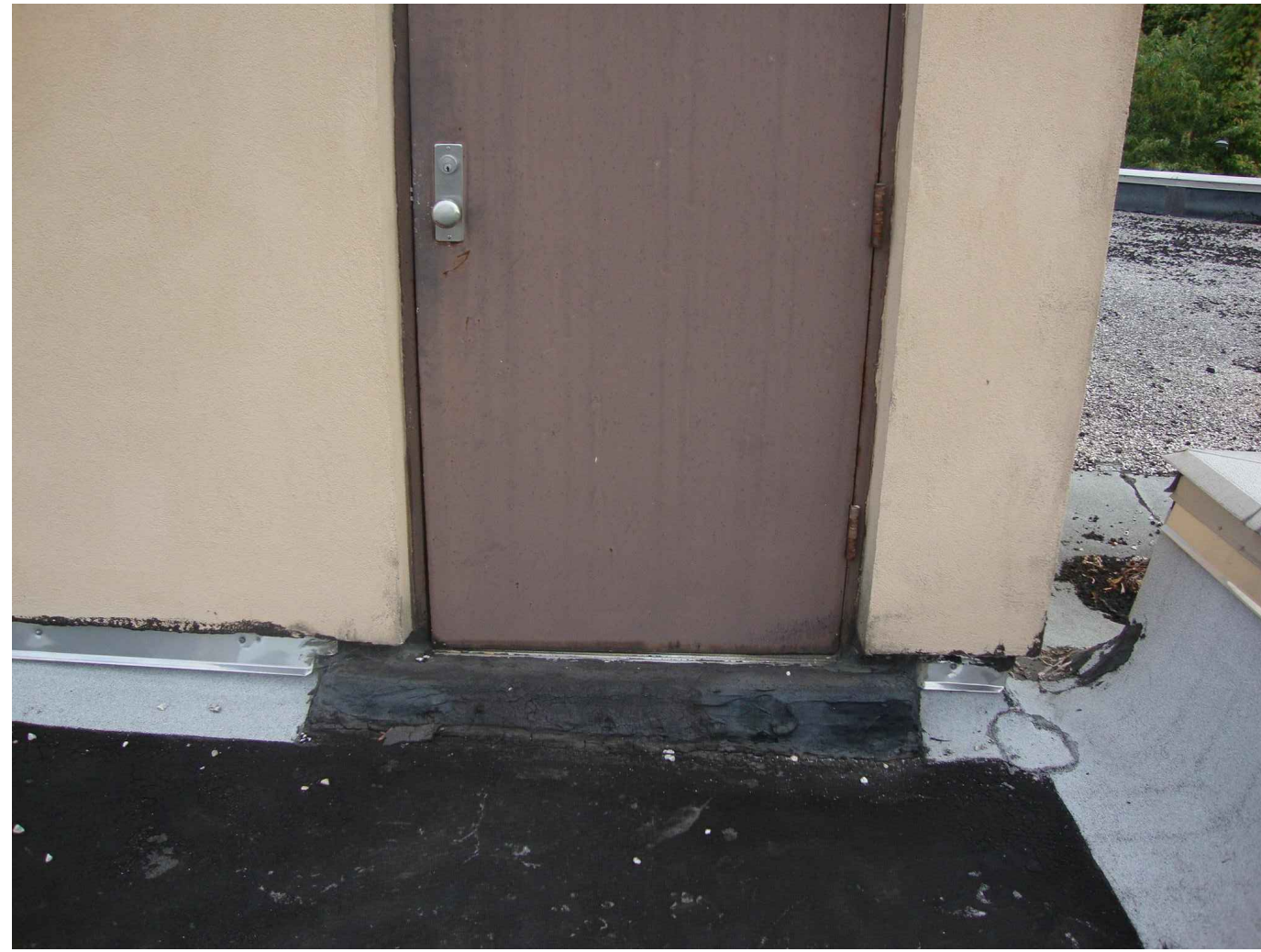
PHOTO # 13 - STAIR TOWER DOOR
