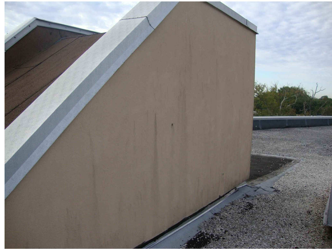
PHOTO # 26 - STAIR TOWER
