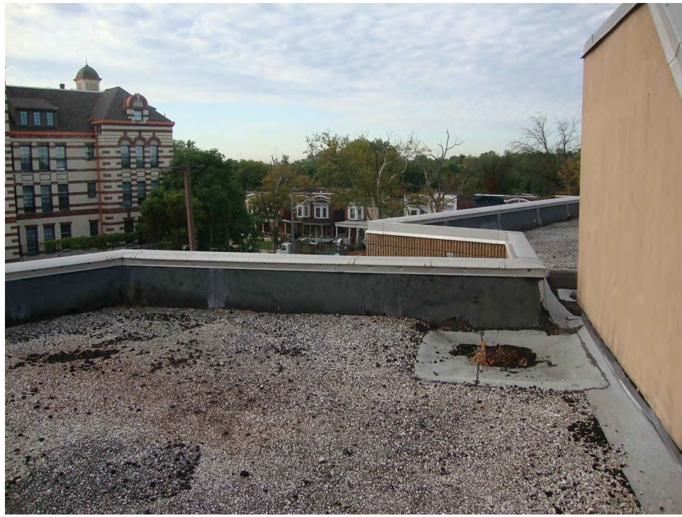
PHOTO # 25 - ROOF DRAIN NEAR STAIR TOWER
