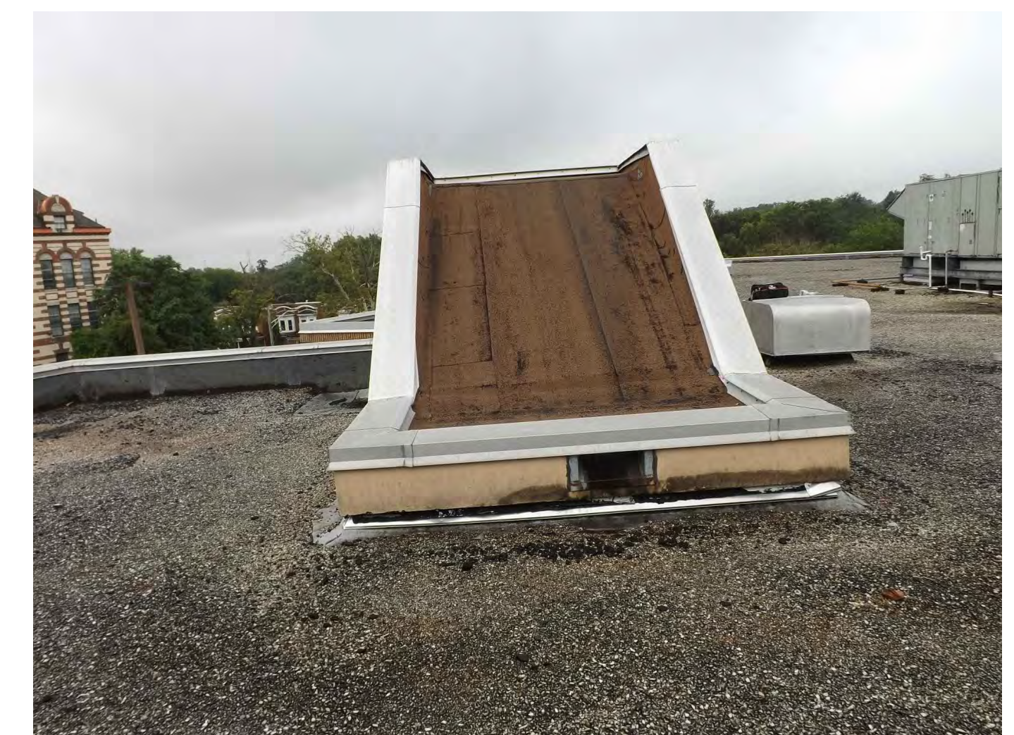
PHOTO # 36 - STAIR TOWER ROOF
