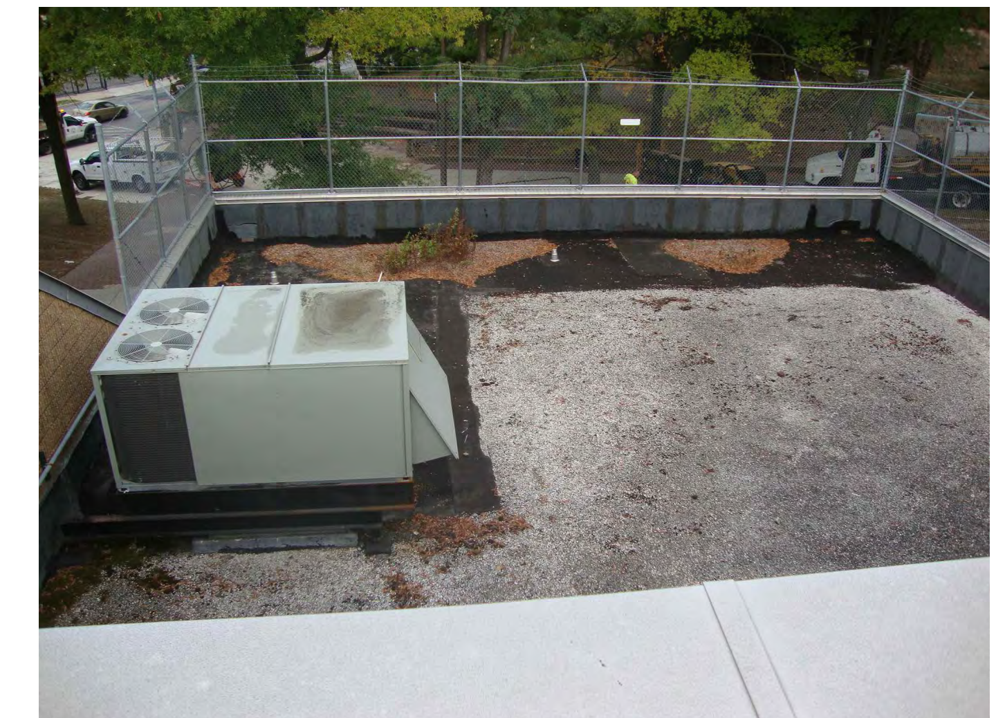
PHOTO # 20 - TERRACE ROOF
