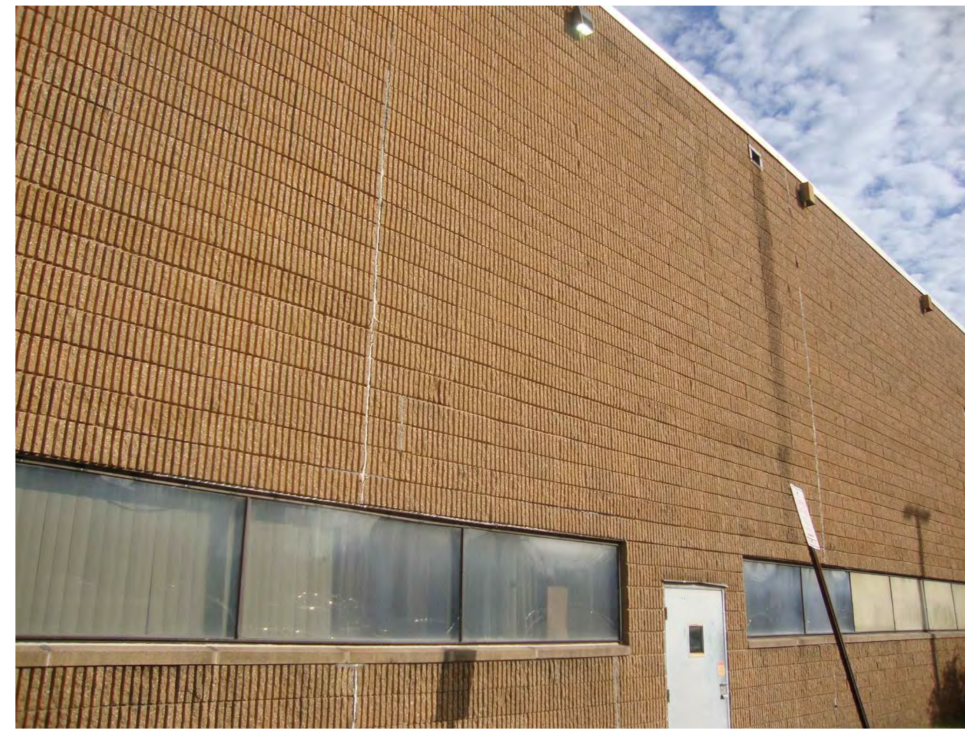
PHOTO # 31 - SPLIT FACE FLUTED BLOCK AT WALL
