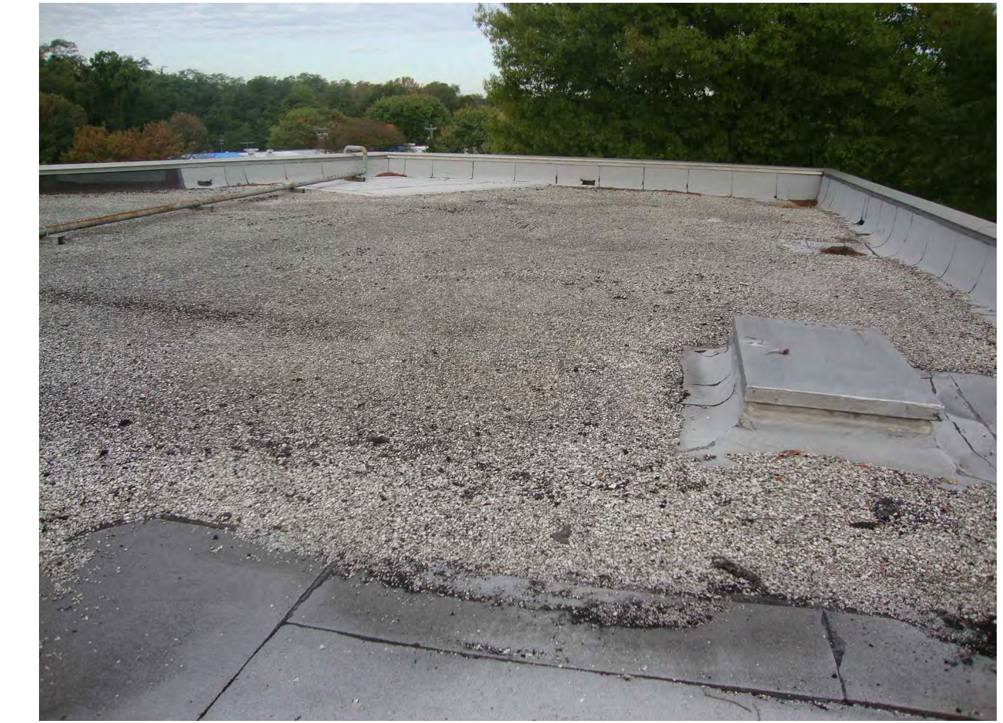
PHOTO # 16 - MAIN ROOF
