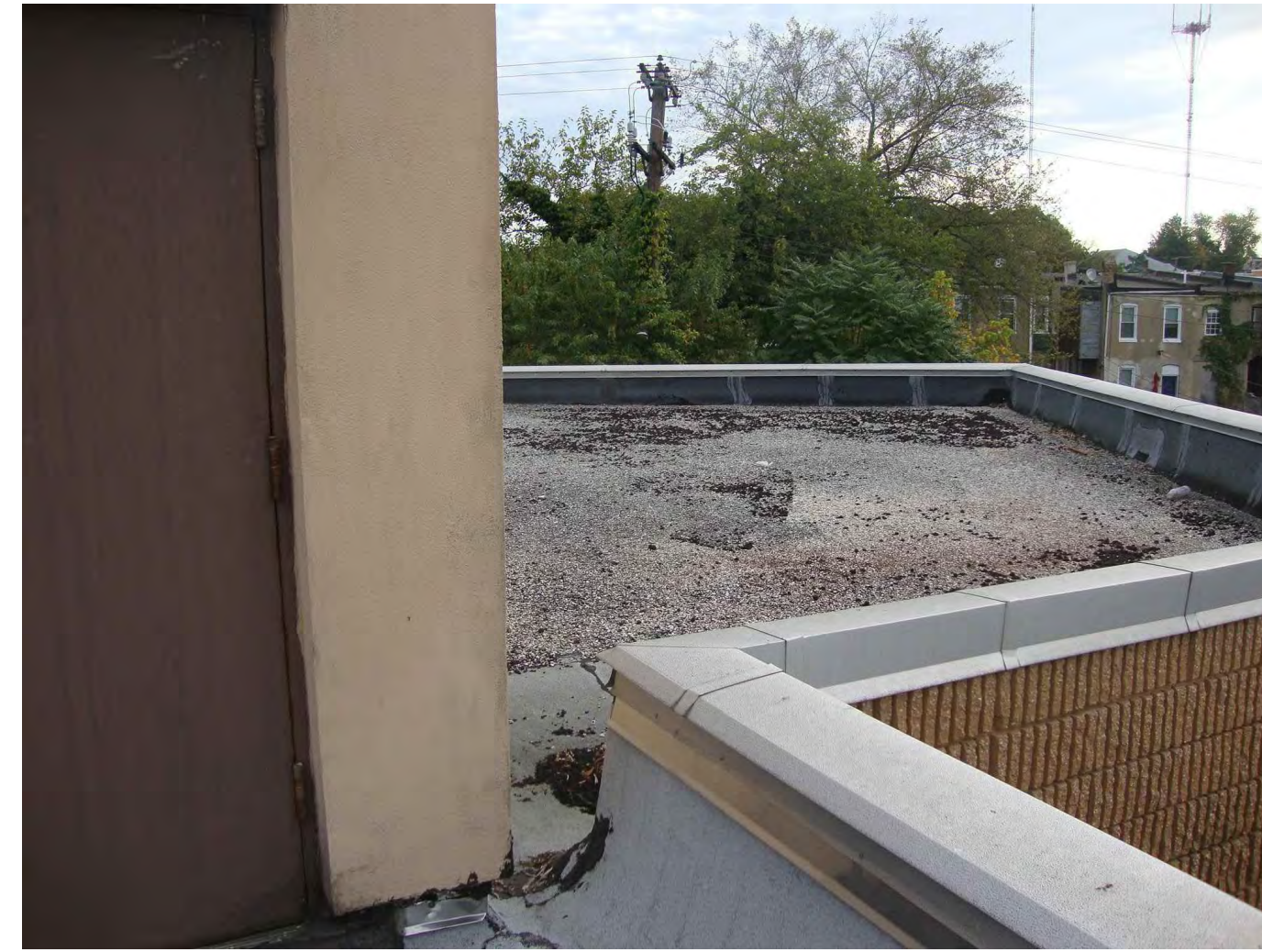
PHOTO # 14 - STAIR TOWER / PARAPET WALL
