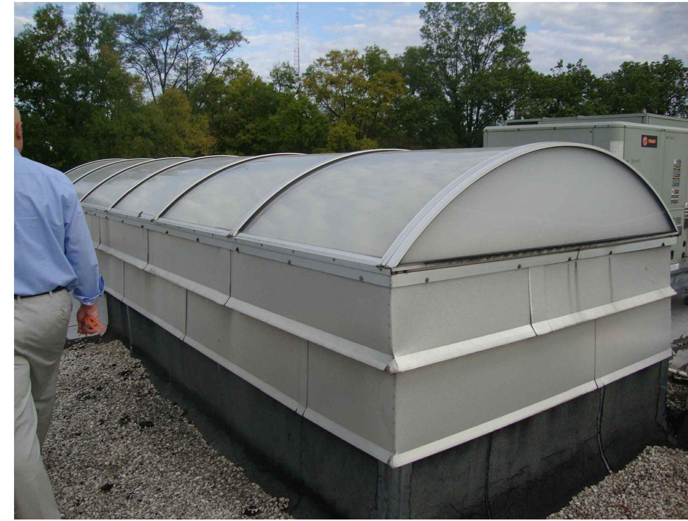
PHOTO # 15 - SKYLIGHT AT MAIN ROOF
