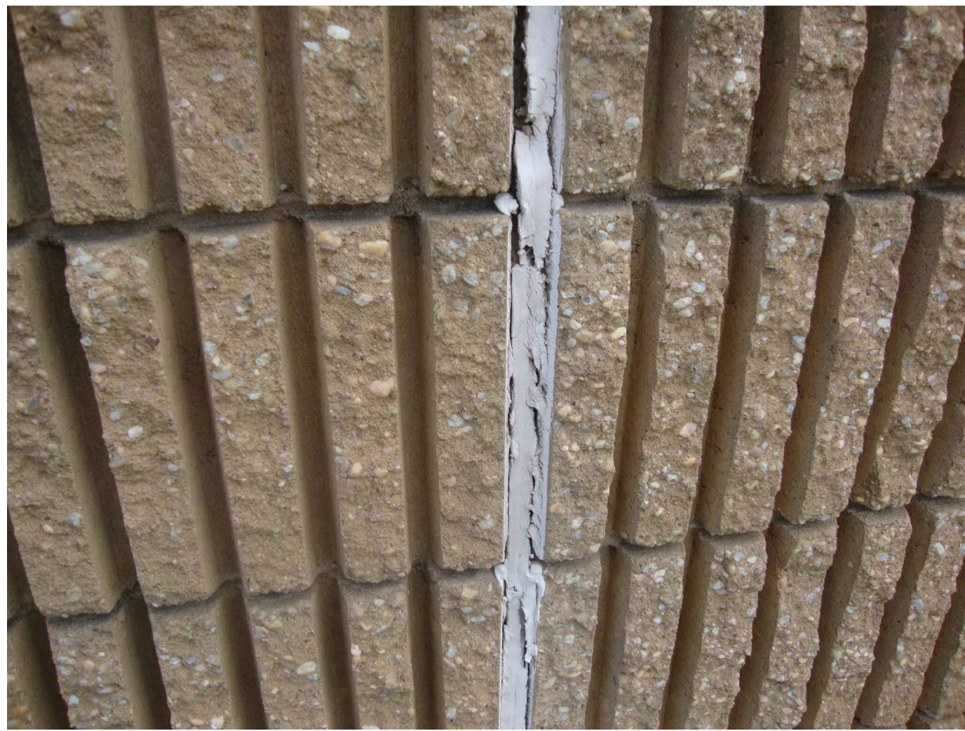
PHOTO # 29 - SEALANT JOINT AT FLUTED BLOCK
