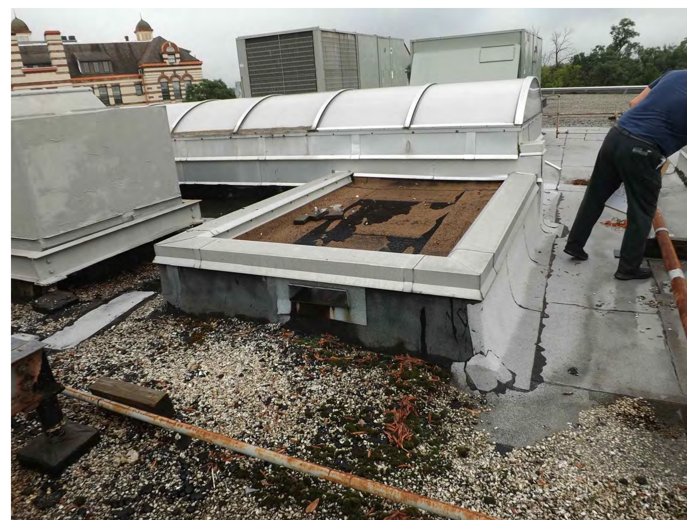
PHOTO # 35 - ELEVATOR ROOF
